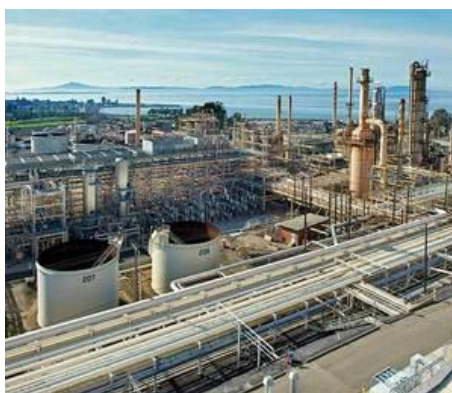
This aging Phillips 66 refinery in Rodeo, California, with access to the San Francisco Bay, is slated to be reconfigured to produce 680 MMgy of renewable diesel, renewable gasoline and sustainable aviation fuel. The project is dubbed Rodeo Renewed. PHOTO: PHILLIPS 66
